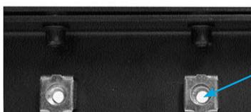
Pre-installed cage nuts
